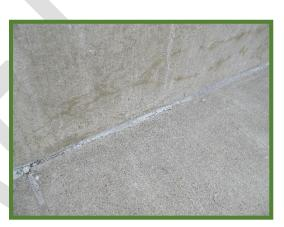
Most of these sealants appear to be very old and are at the end of their useful life. The typical service life for joint sealants is 7 to 10 years, especially at the roof level. Sealants should be repaired to prevent the infiltration of moisture and chlorides into the structural elements below and to prevent leaking onto vehicles and pedestrians at the Lower Level.
